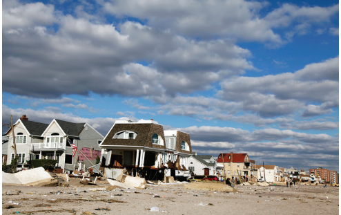
Thousands of homes were destroyed by Hurricane Sandy
